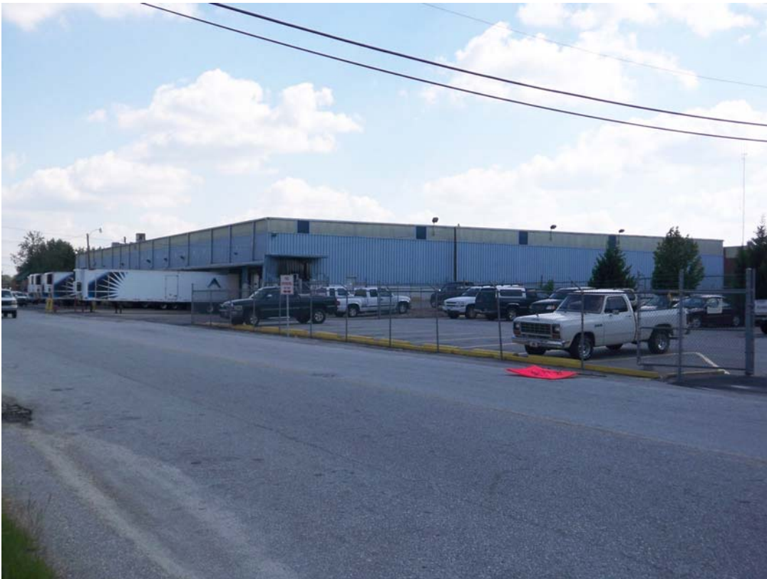
US Food Service Building – 215 Commerce Drive
